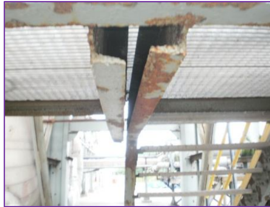
Scaling and pitting on steel members
