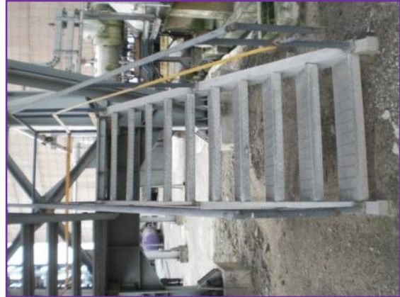
Corrosion, scaling and pitting on weld connection and steel members
