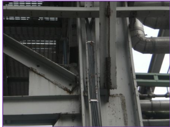
Crack on top layer of RCC pedestal / Nut bolt missing and insufficient welding
