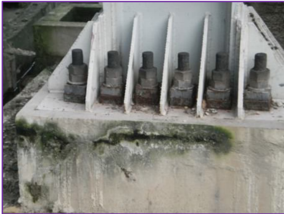
Crack on top layer of RCC pedestal / Nut bolt missing and insufficient welding
