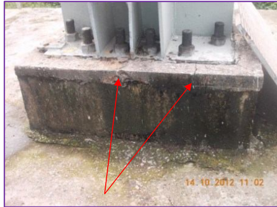
Crack on top layer
