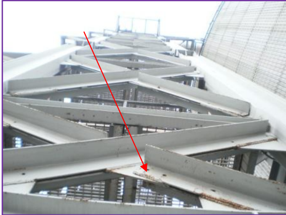
Corrosion, scaling and pitting on weld connection and steel members
