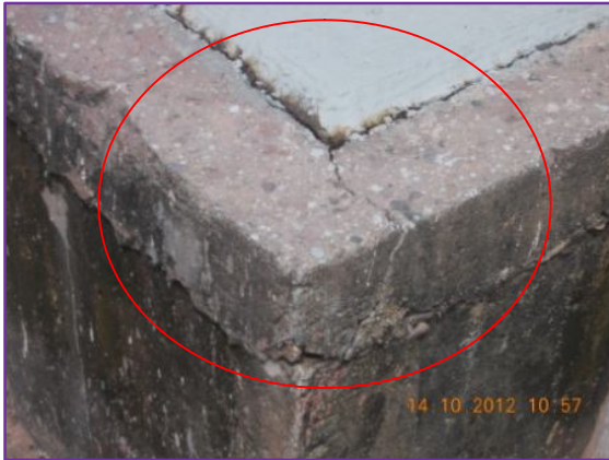
Crack on top layer
