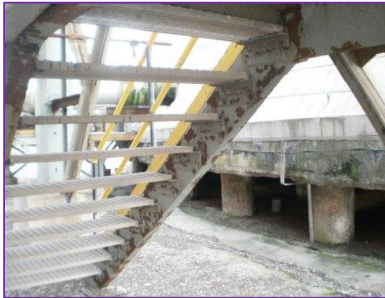
Scaling and pitting on steel members
